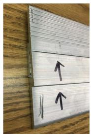
9) There are tabs on the bottom of your sign for you to add additional wall anchors, so the sign can't be lifted off of the french cleat. Drill and insert the wall anchors here as well.
