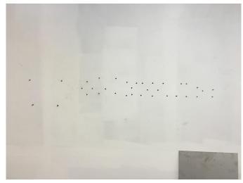
Step 4 - Insert pieces with all thread on the back, with spacers, into the drywall, press them into place. Sometimes you have to lightly tap on the face of the letters to get the all thread to fit into the drywall.
