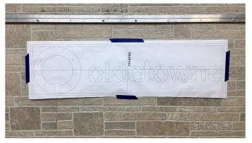
Step 3 - Drill pilot holes through all of the areas indicated on the template, after drilling pilot holes, remove the template and drill  $\frac{1}{8}$  or  $\frac{9}{64}$  holes for the 6-32 thread and  $\frac{3}{32}$  for the 4-40 thread.
