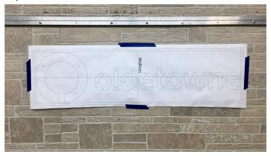
Step 3 - Drill pilot holes through all of the areas indicated on the template, after drilling pilot holes, remove the template and drill  $\frac{1}{8}$  or  $\frac{9}{64}$  holes for the all thread.
