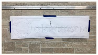
Step 2 - Drill pilot holes through all of the areas indicated on the template, after drilling pilot holes, remove the template and drill holes to close as possible to the same size as the all thread. This is ideal to ensure a tight fit into the wall surface. (Depth needs to be deep enough so that the stem with spacer is flush with the wall).
